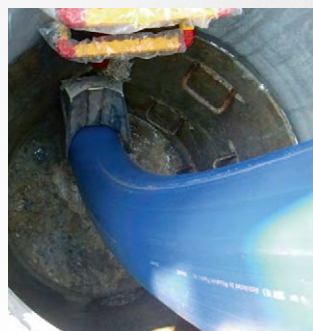
Japan, Osaka, DN250, Trinkwasser
